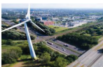
Infrastructure and climate change an overview
